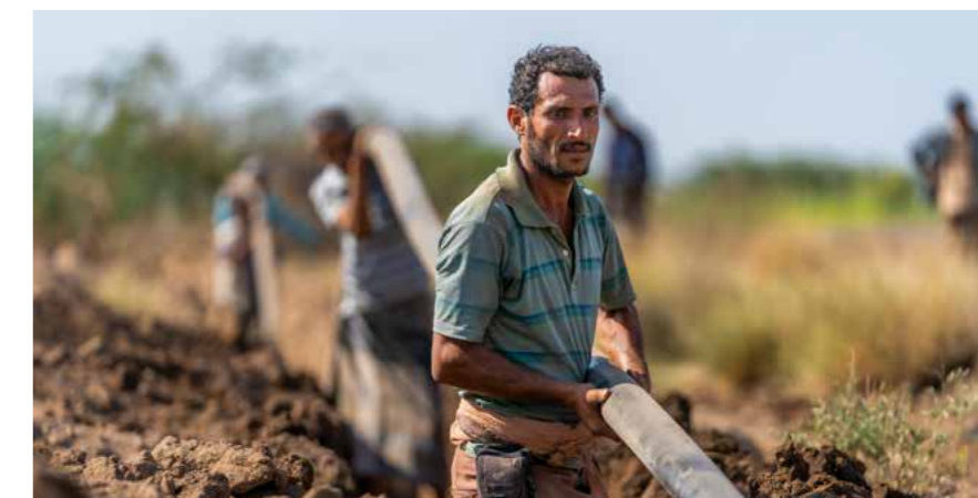
In the south of Yemen, we concentrated on repairing drinking water sources. Photo: PIN archive
